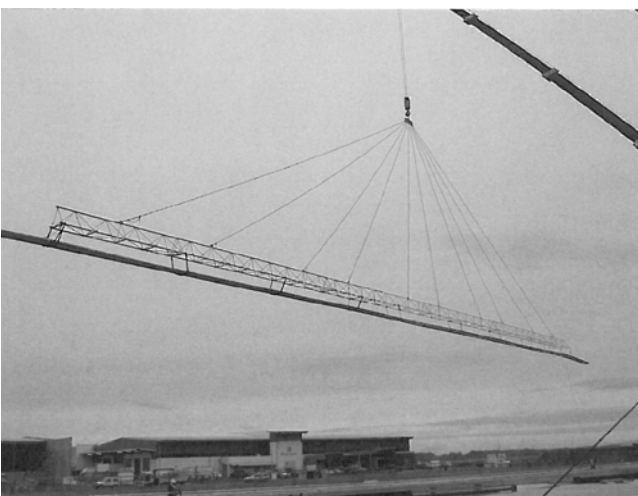
Dimondek® 630 65 1m sheets on Lifting Boom
