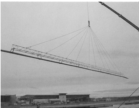
Dimondek® 630 65 1m sheets on Lifting Boom
